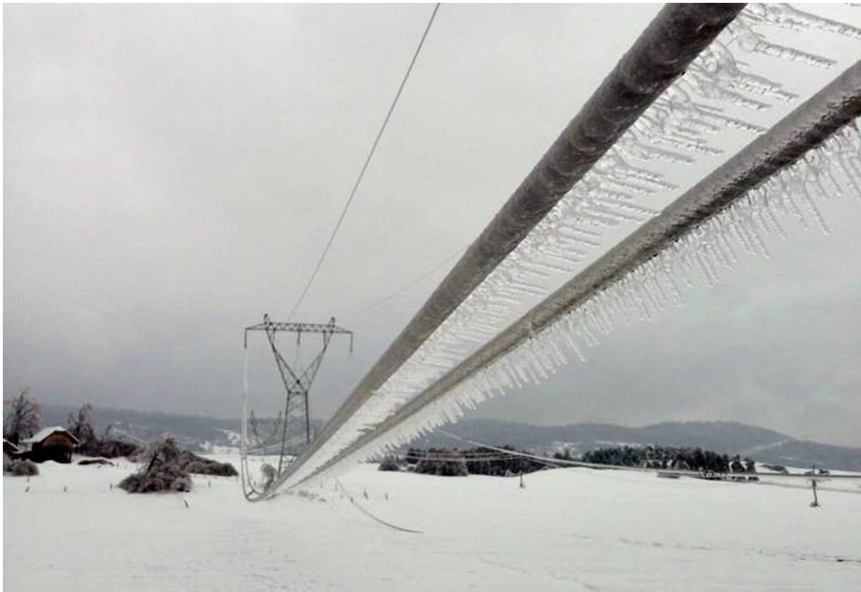
Figure 1: The image shows an overhead powerline that collapsed due to extreme icing. This event triggered the creation of software for thermal management which evolved into DiTeR. Eles d.o.o., February 2014.
